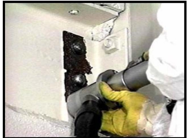
**CORNER-CUTTER<sup>®</sup>** scarifies inside corners, outside edges, and flat surfaces!
