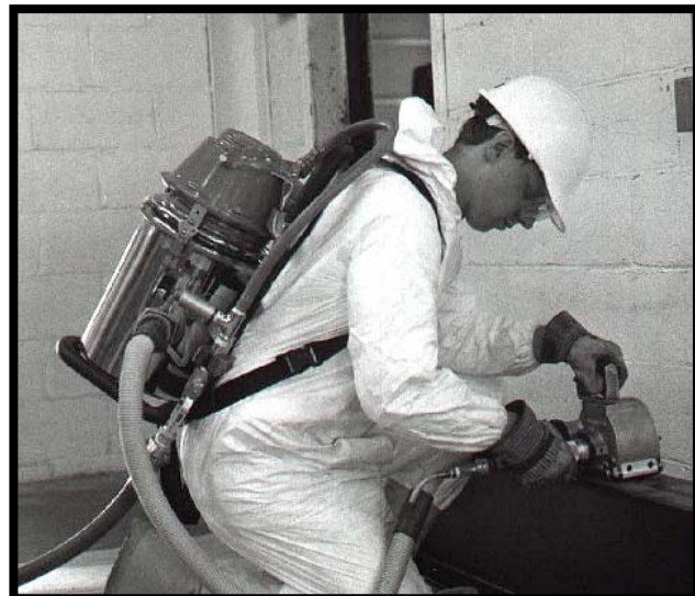
The COMPACT-VAC collects all dust and debris as the ROTO-PEEN Scaler prepares steel, concrete, brick and wood surfaces at a nominal rate of 45 sq. ft./hr.
